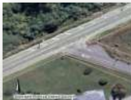
Pre-works: No turn-bay!
